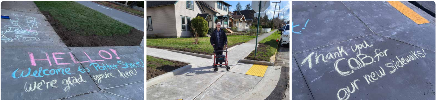
The YNA would like to thank the City of Bellingham for the new well-constructed sidewalks on Potter Street, across the heart of our neighborhood. We are grateful for the hard work and dedication to making the York neighborhood accessible to all community members!
